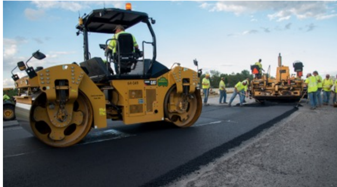
Example of roadway paving
