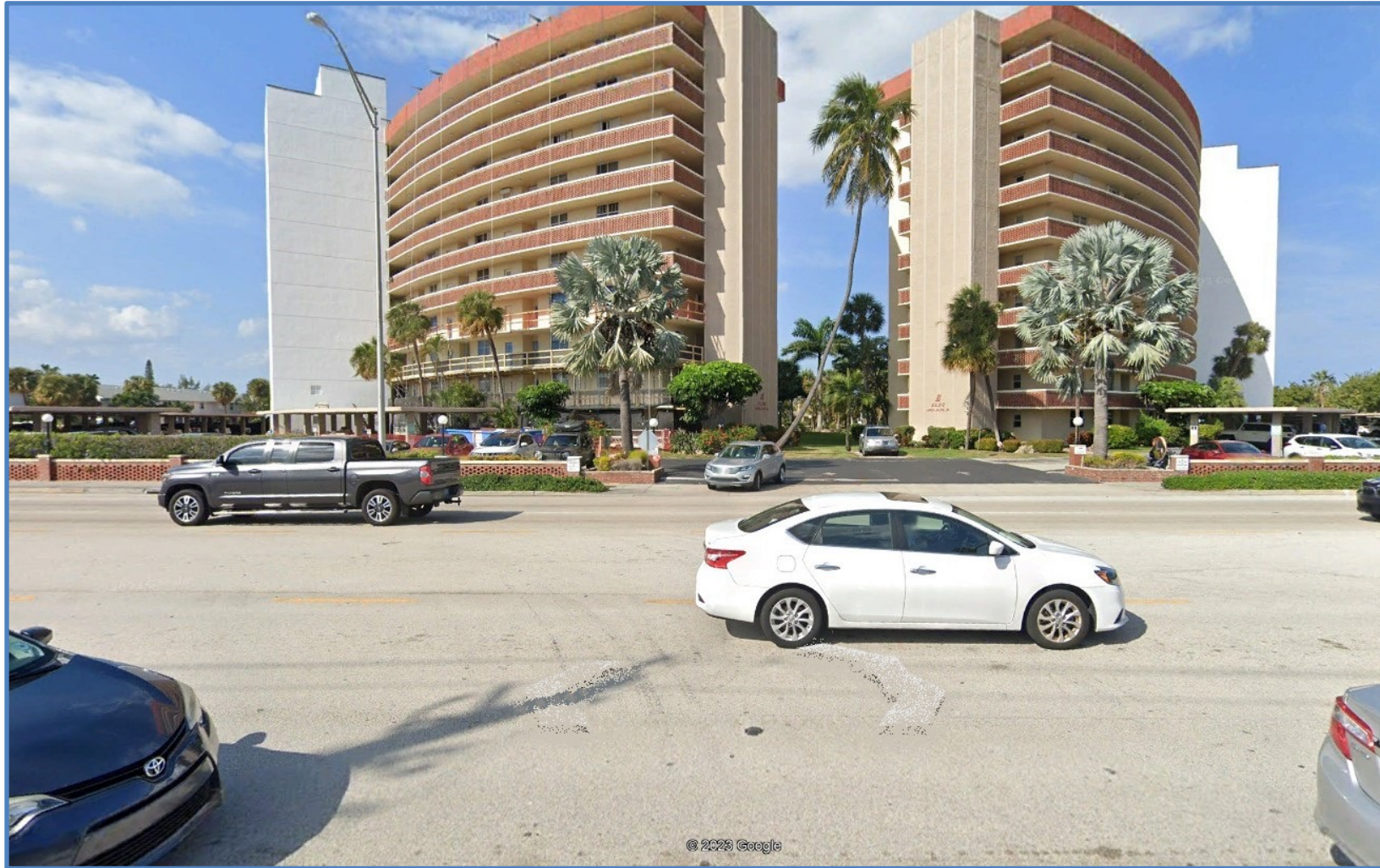
At NE 28 th Avenue Median Opening Location Looking North
